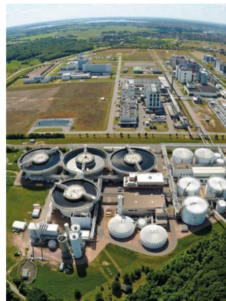
Joint sewage treatment plant, in background: Bitterfeld-Wolfen Chemical Park (Source: GKW).
