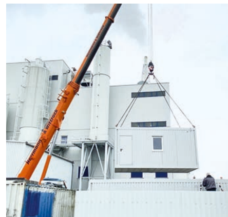
Container setup in December 2021.
